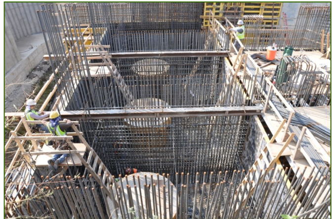
Shown is the Enhanced Nitrogen Removal Facility under construction.
